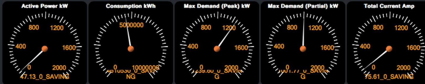
Chiller 01 Power Data
